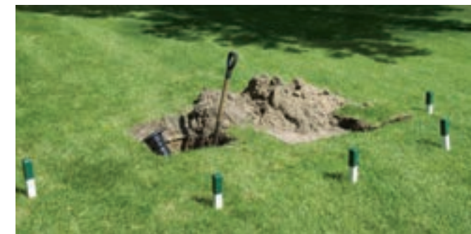
Mark off repair areas.
